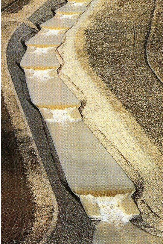
Figure 6 – Providing the energy of the water is sufficiently absorbed at the gabion weir it is possible to opt for a grassed channel below the weir (Designed and built - DFA, 2002).
