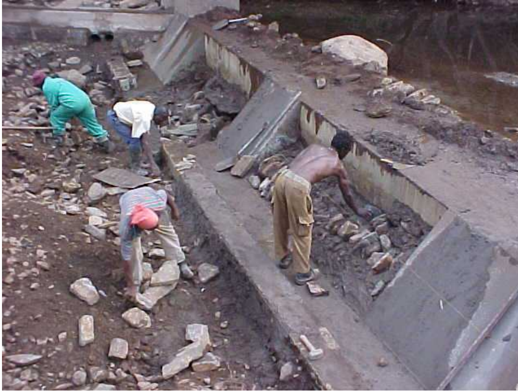
Figure 7 – Where ground is well consolidated it may be cost effective to construct the weir from a more rigid system such as random-rock-masonry as shown here. Much of the ground from which the re-engineered spillway is to be constructed is either undisturbed or well compacted, making this type of construction an option in the final design, if better suited than gabions. This diversion weir is situated in a gorge that has a 130km 2 catchment. (Designed and built – Dams for Africa 2003/4).
