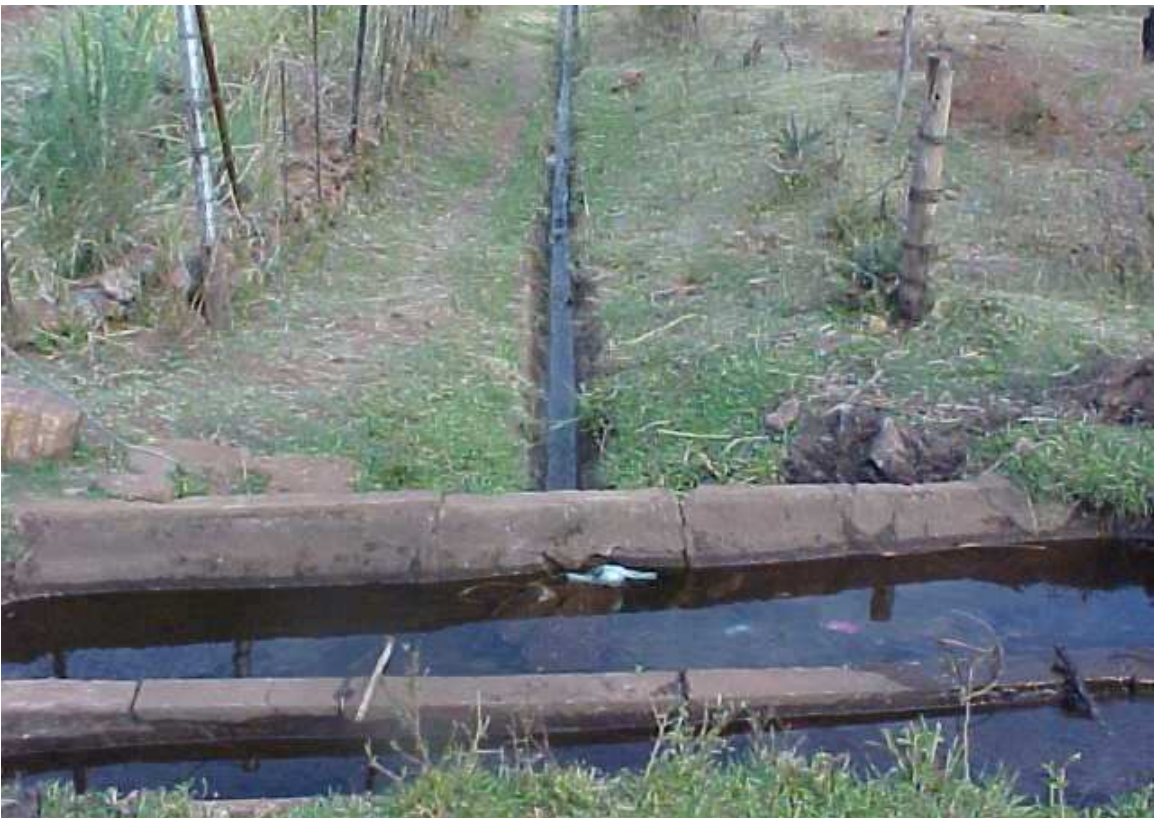
Figure 9 – View of the first secondary canal coming off the first gate
