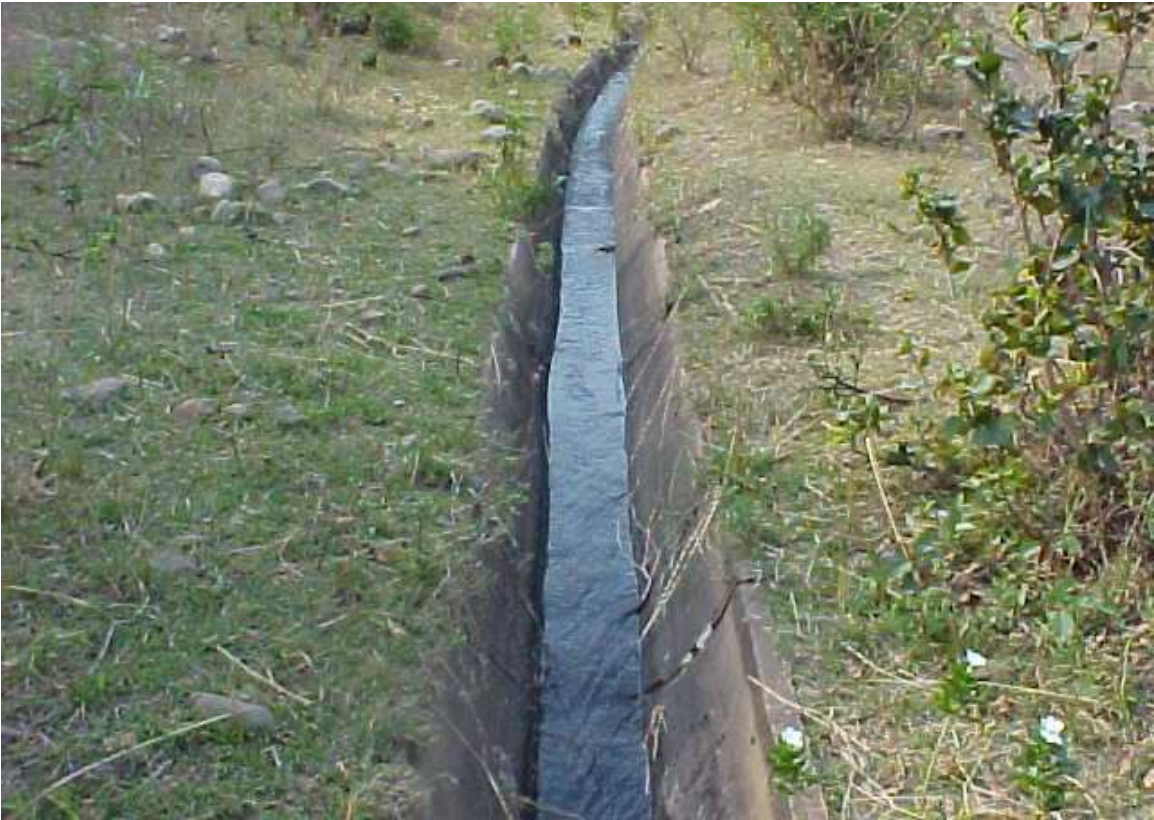
Figure 8 – View of principal canal
