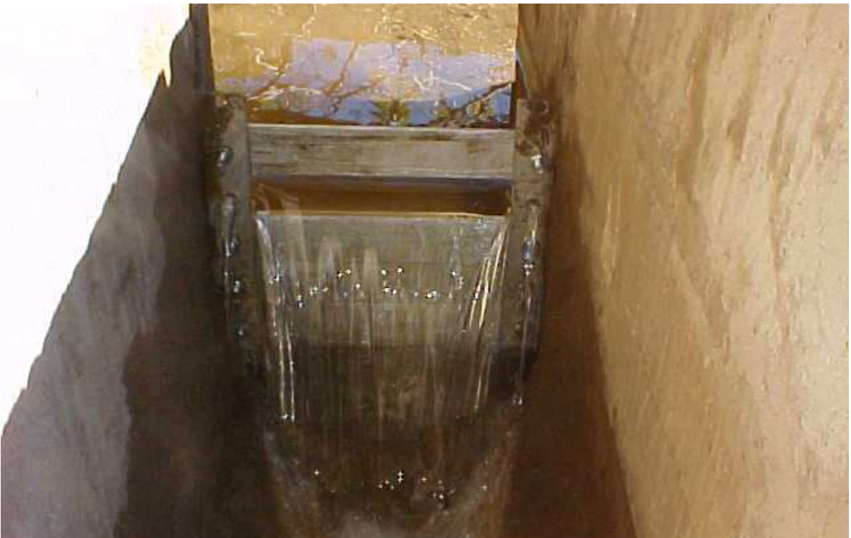
Figure 7 – A simple sluice gate, made from removable steel plates to allow adjustable flow.
