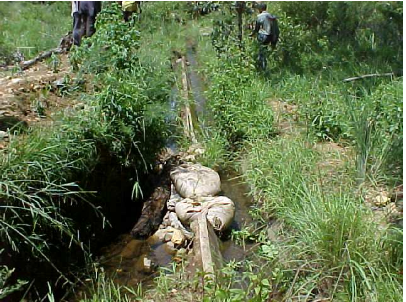
Figure 3 : The low level of the water in the reservoir results in minimal water flowing in the canal. An unsuccessful attempt to bring in water from the side was made.
