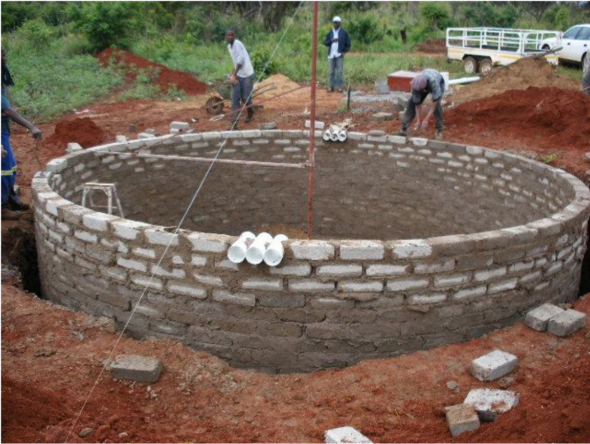
Figure 3 – A standard dam under construction
