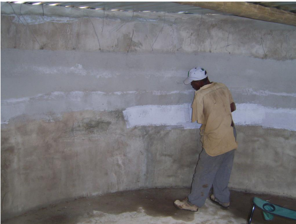
Figure 4 – A view inside with the waterproofing operation underway
