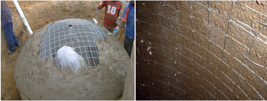
Figure 2 – Ferrocement consists of chicken mesh fastened to a wire frame (see bottom left), and to this a cement-sand mortar is applied in two stages. On day one a thin skin of about 1cm thick is applied (see top left). Bottom right indicates how the mortar has only just moved past the chicken mesh. By day two the thin mortar skin will have stiffened the shell sufficiently for a final application of 2cm on the inside (see top right), followed by a similar application on the outside.
