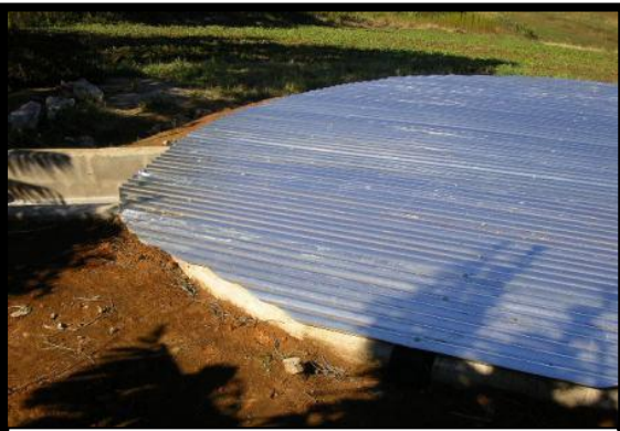
Underground RWH dam in the backyard, safely roofed so that no child can fall in
