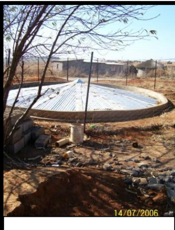
Underground RWH dam. Note interesting sunken roof which catches water falling onto its own roof
