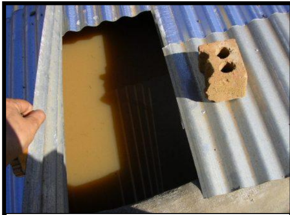
RWH dam - full of water! The trap door in the roof must keep children out, yet provide access to clean out the tank.
