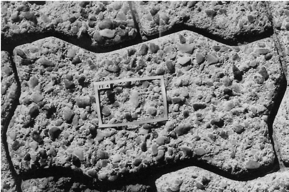
Figure 12.2 Highly exposed aggregate particles of blocks in service for 8 years at factory entrance. They are usually the result of either insufficient water or binder content.
