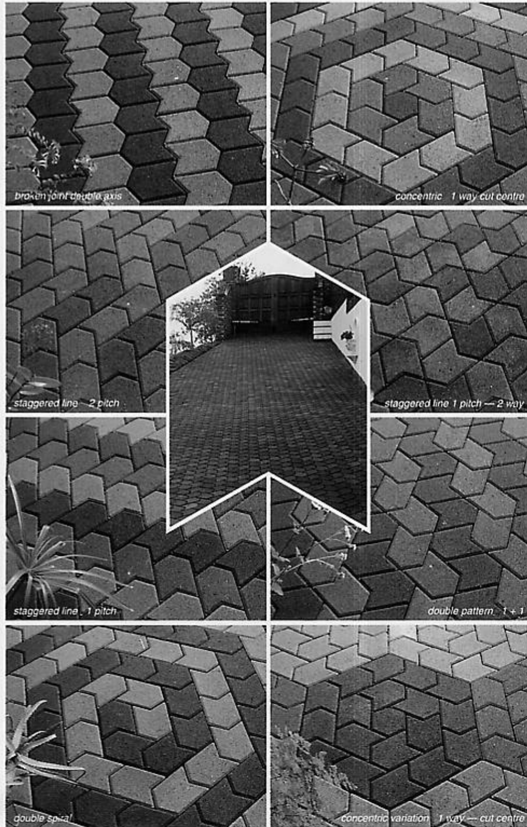
Figure 2.1 Various laying patterns from one block
