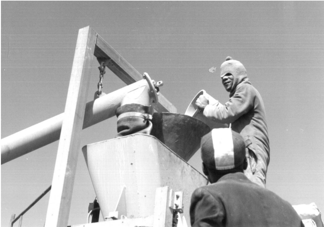
Figure 3.4 Binders of known quality were poured into the top of the cement scale from bags
