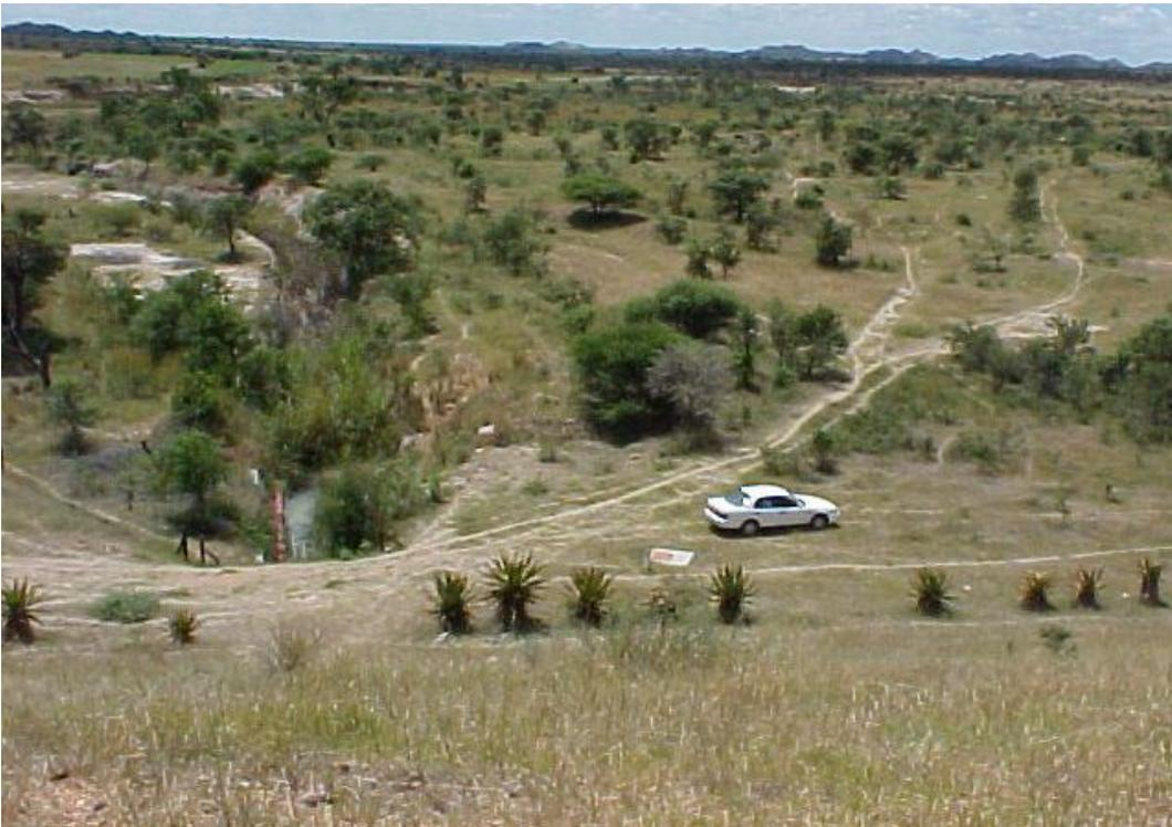
**Figure 6** – Downstream view from the top of the dam, showing irrigable lands to the right of the stream. The pipe going to the purification plant may be seen exiting the delivery tunnel.
