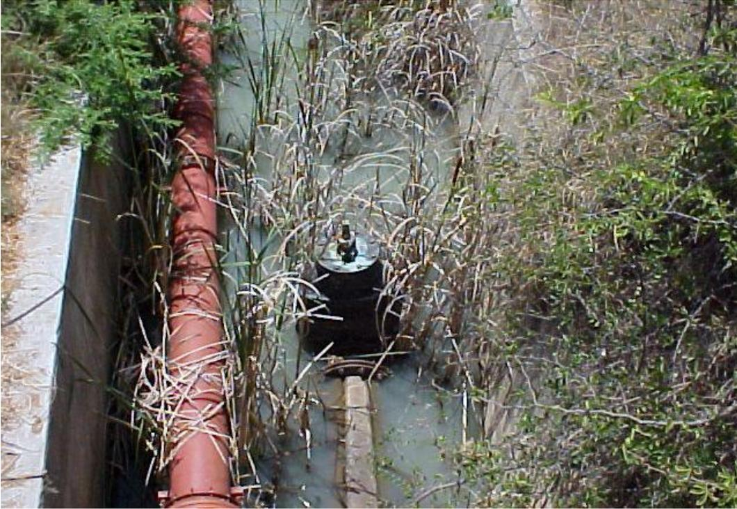
**Figure 5** - Pipes on the downstream side exiting the delivery tunnel. The pipe on the LHS delivers water to the water purification plant, while the RHS pipe terminates as shown
