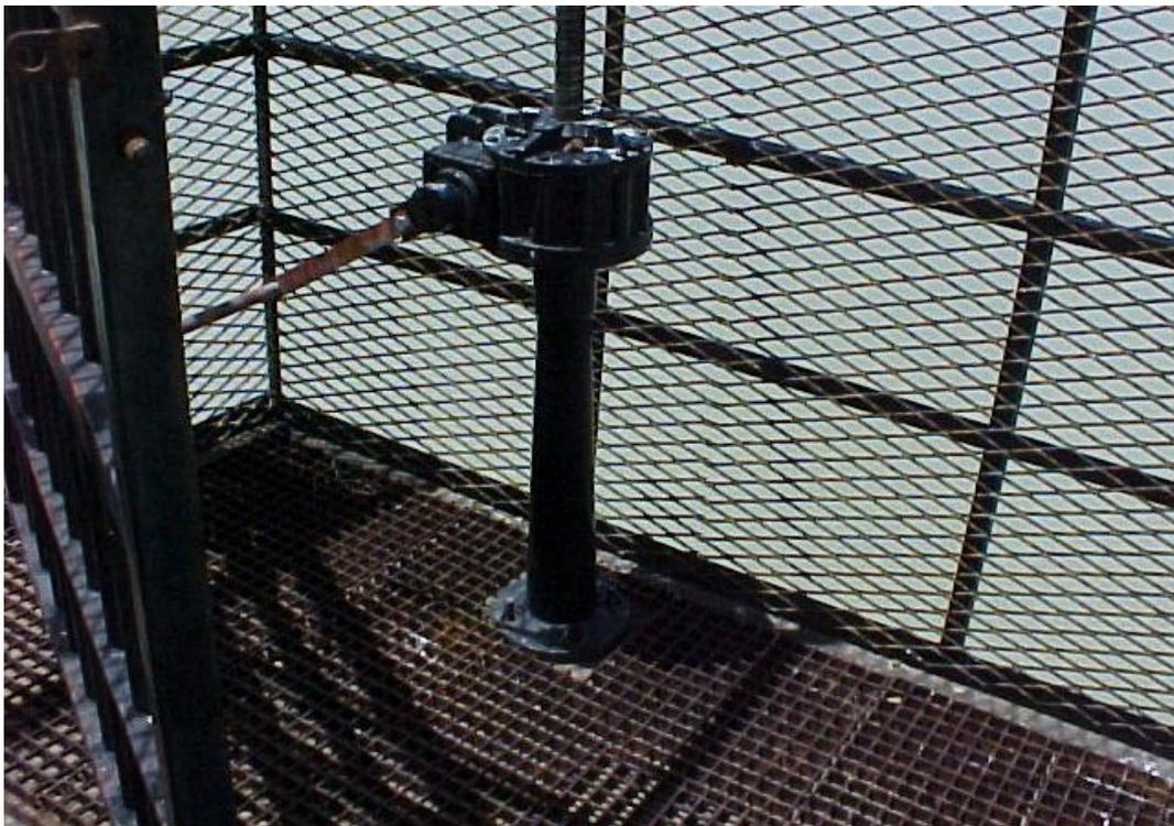
**Figure 4** – Each pipe in the intake-tower/delivery-tunnel begins with a valve that can be opened or closed by means of a remote handle
