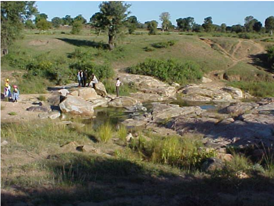
Figure 4 – Overview of the site where the second dam is proposed - seen from the left flank, showing exposed rock-bed and relatively steep flanks.
