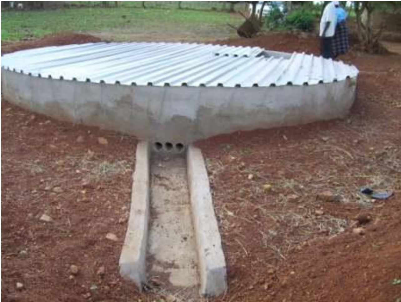
Figure 6.3 – Standard Overflow structure
