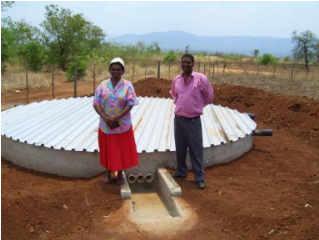
Figure 6.2 – Standard Inlet Structure
