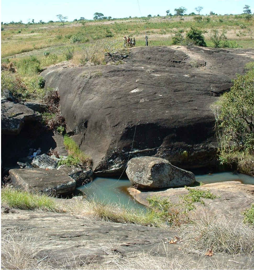
● Figure 5 – Proposed site for RRM arch. The upstream end is on the left of the photo. The rock appears to be almost free from fractures, and the opposing abutments appear to be suitably angled for the construction of an arch dam.
