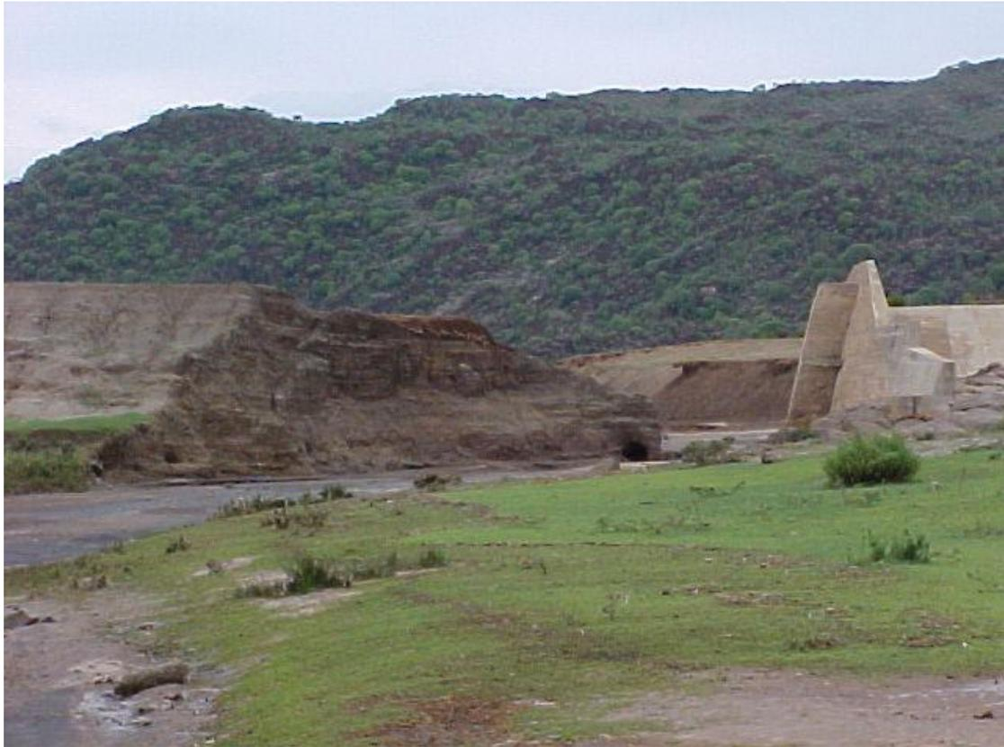
**Figure 1** – View of breach in dam
