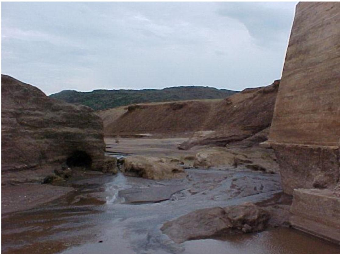
**Figure 2** – Downstream view showing the degree of sedimentation and the incorrect slope in the bottom section of the concrete abutment
