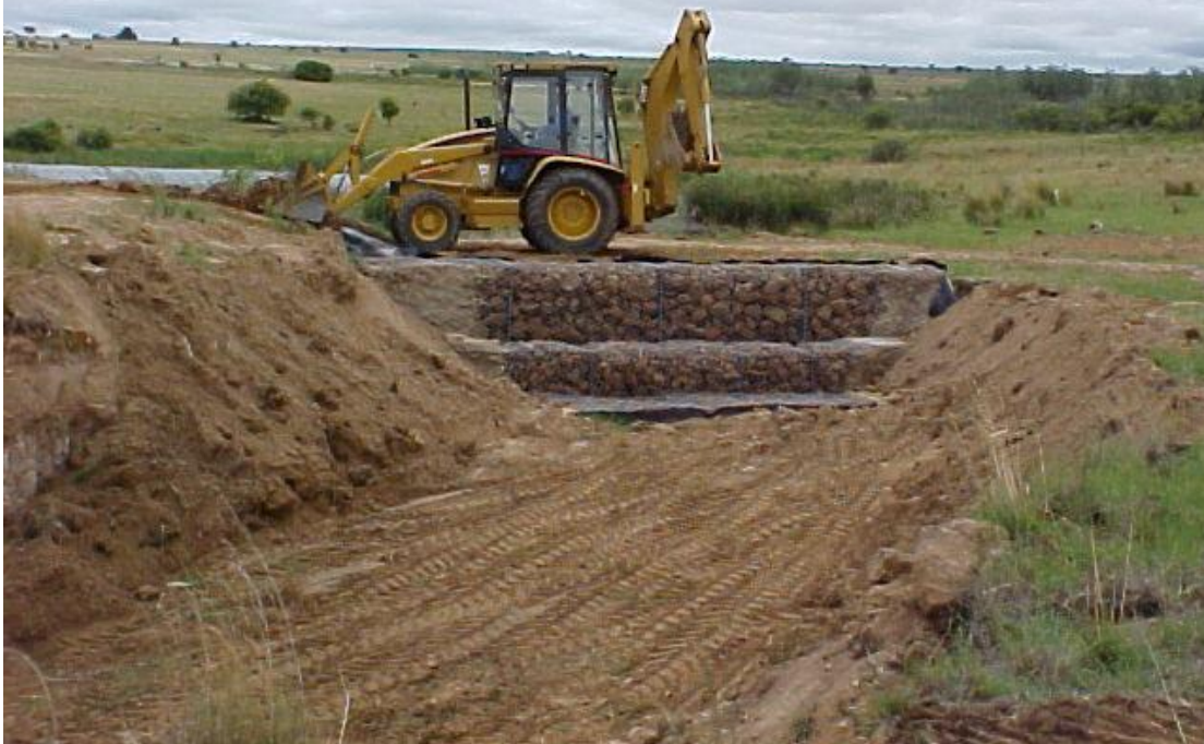
Figure 6 – Providing the energy of the water is sufficiently absorbed at the gabion weir it is possible to opt for a grassed channel below the weir (Designed and built - DFA, 2002).
