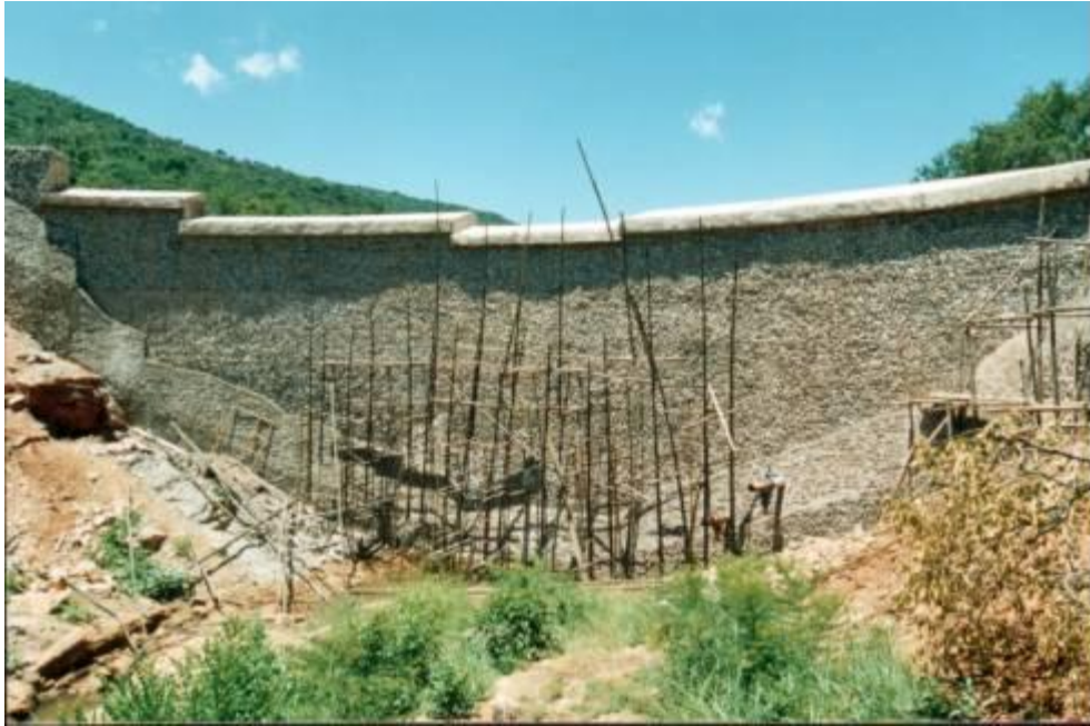
Figure 1-4 A cantilever-arch dam made from rock-masonry. The wall is 17m high with a 28 m radius.
