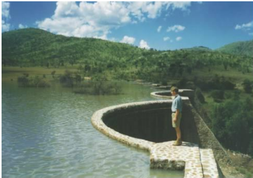
Figure 3 Buttressed multiple arch-dam made from rock-masonry, Pilanesberg Nature Reserve
