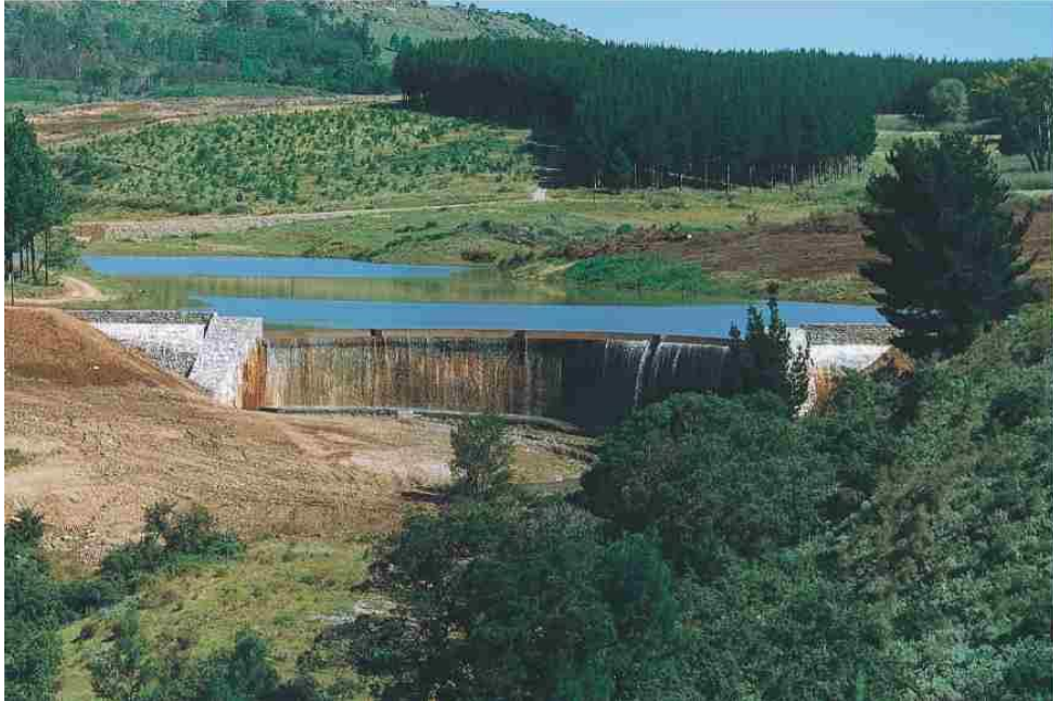
Figure 2 Example of an arch dam made from rock-masonry, Hogs back.
