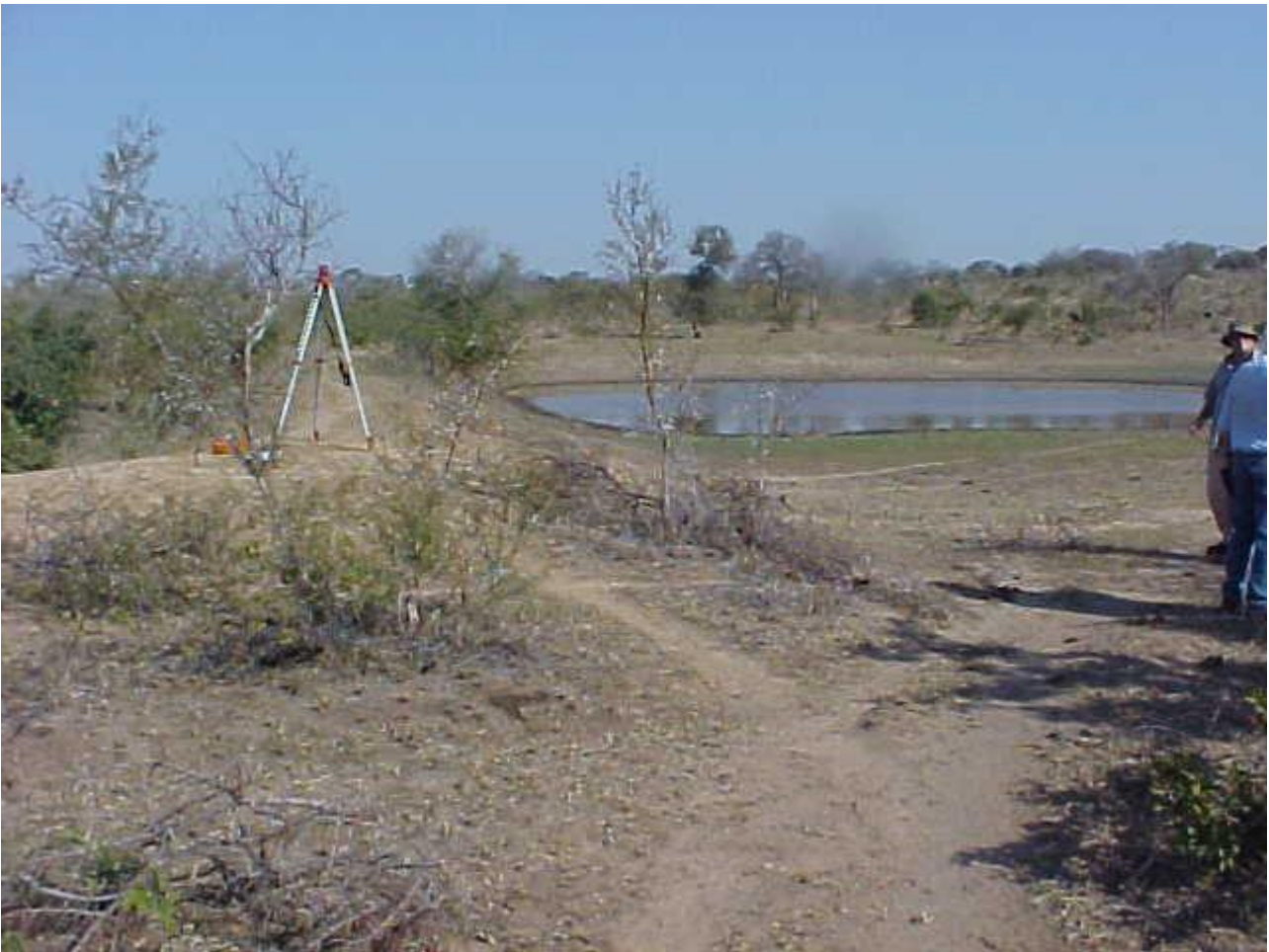
Figure 2 – A view of the Newington C dam. This dam still has approximately 700mm water left in it. The photograph is taken from the start of the spillway, and the tripod represents the start of the embankment. This dam is estimated to have a depth of 2,6m when full, which explains why there is still some water left in it. (However, it is likely to be almost dry by the time the November rains arrive).
