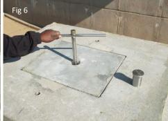
It may be see that the lid is only half the depth of the seat, but what it lacks in thickness it makes up for in reinforcing, as indicated in figure 8, where the volume of reinforcing exceeds 5% (vol/vol), making the lid extremely strong and chisel resistant.
