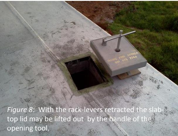
Figure 8: With the rack-levers retracted the slab-top lid may be lifted out by the handle of the opening tool.
