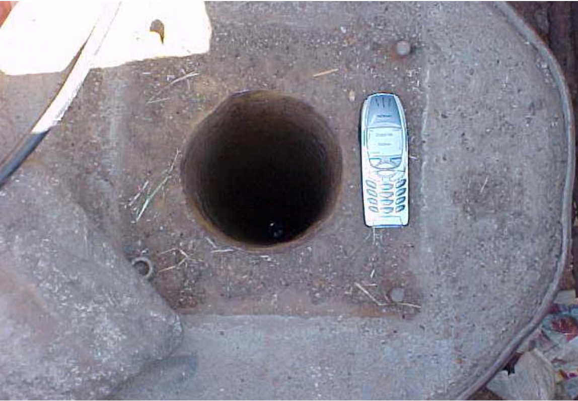
Figure 2 – View of existing borehole
