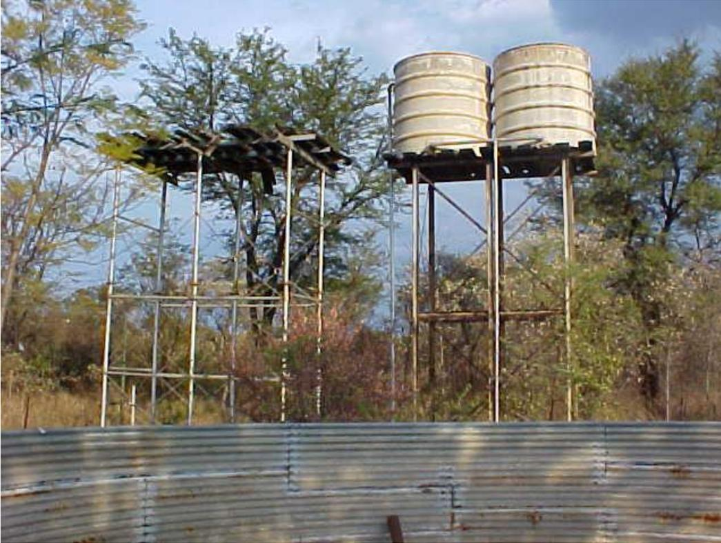
**Figure 5** – view of existing 5000 litre tanks and vacant tank stands
