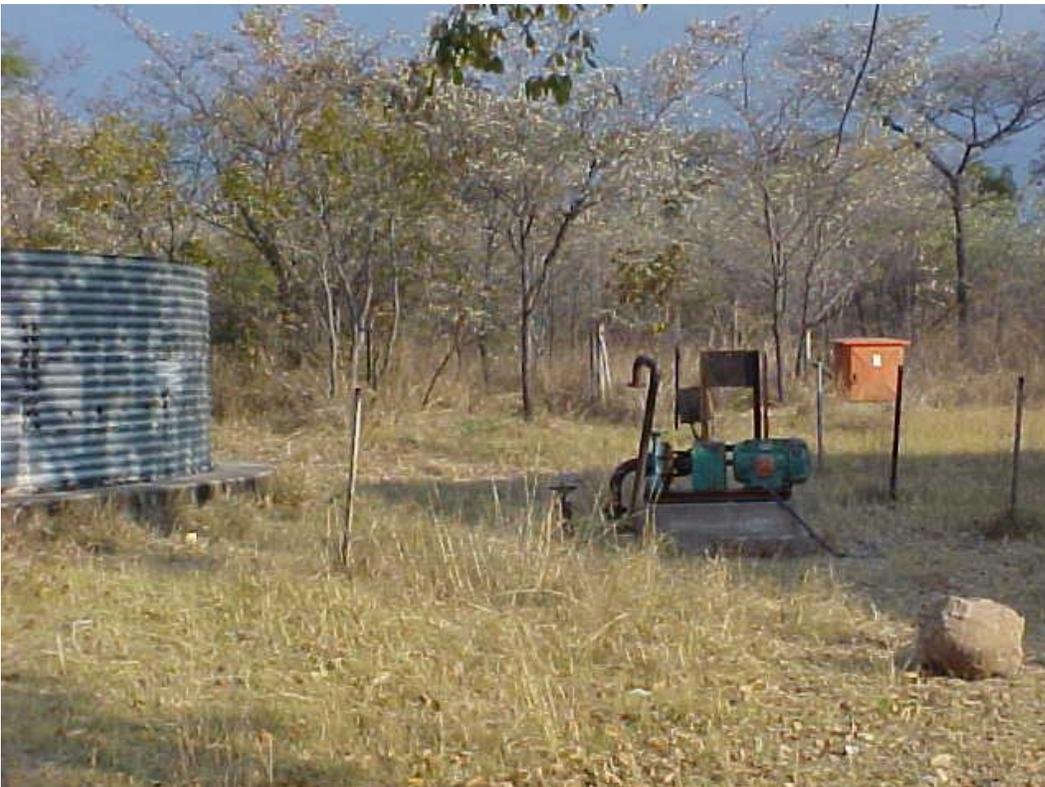
**Figure 6** – view of old centrifugal pump with reservoir on the left and electrical distribution board in the background
