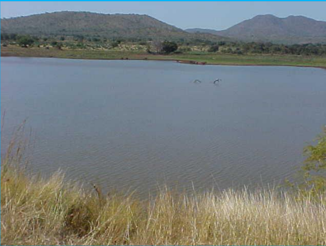
Figure 3 – View across the dam from the embankment
