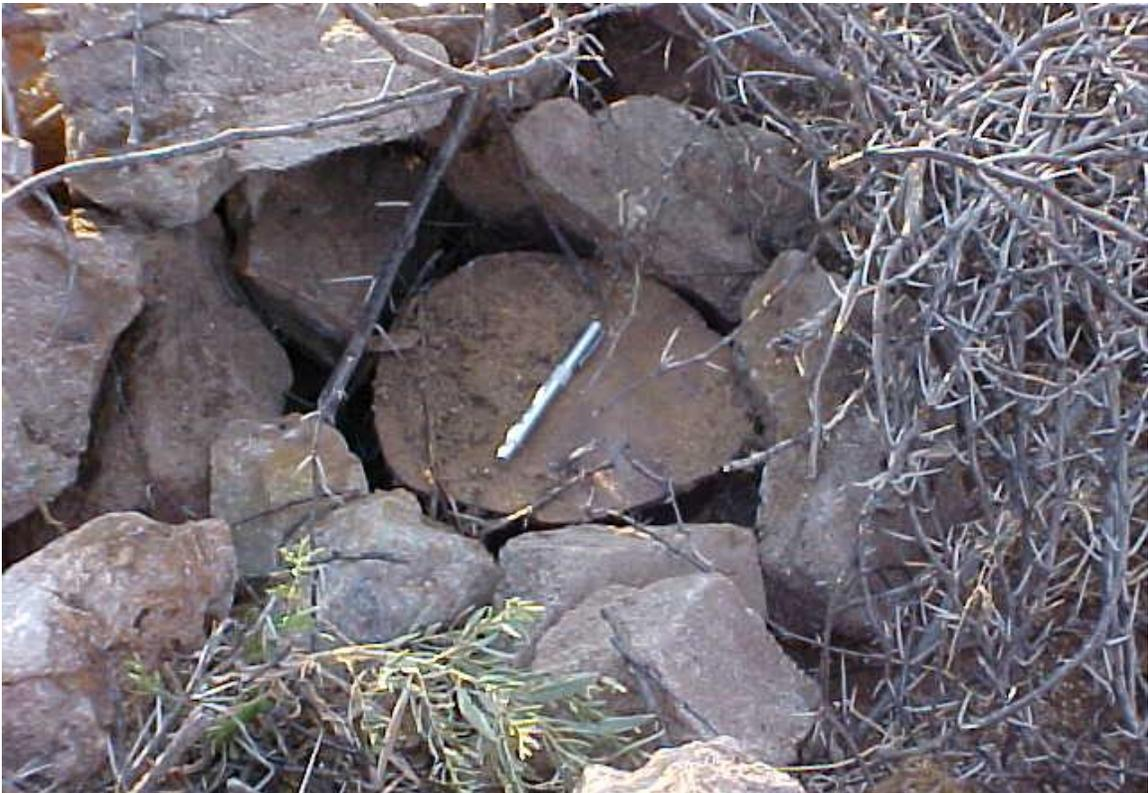
**Figure 2** – The steel casing of the borehole has been sealed off
